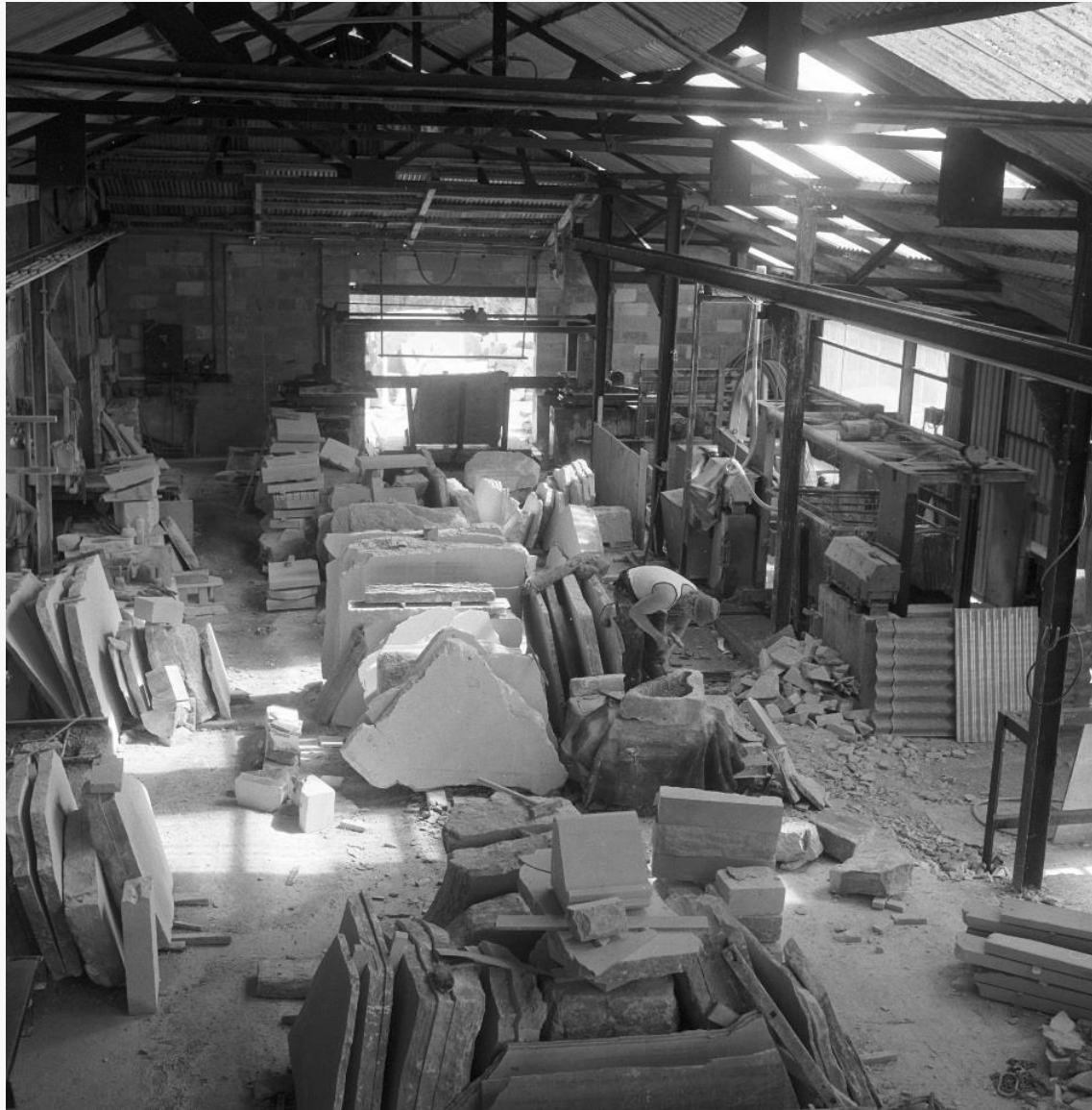
Masonry workshop, interior. 1986
