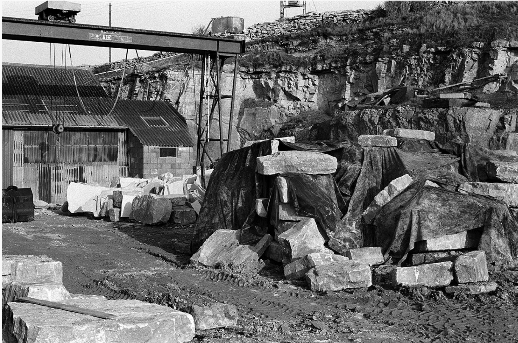
Pond Freestone block protected to prevent frost damage, 2006
